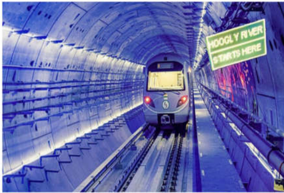
Fig 7. East West Metro Tunnel [18]
