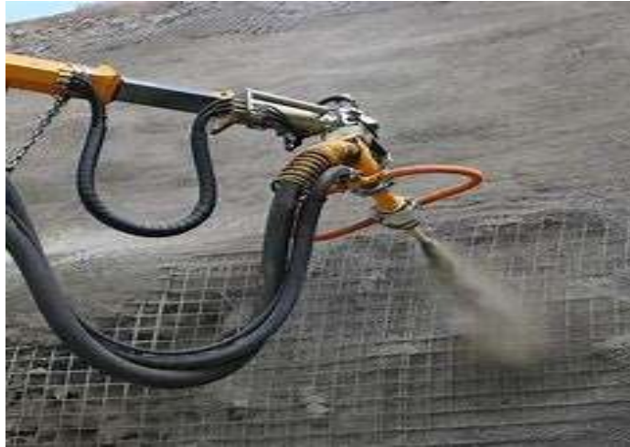
Fig No. 4. Shotcrete
